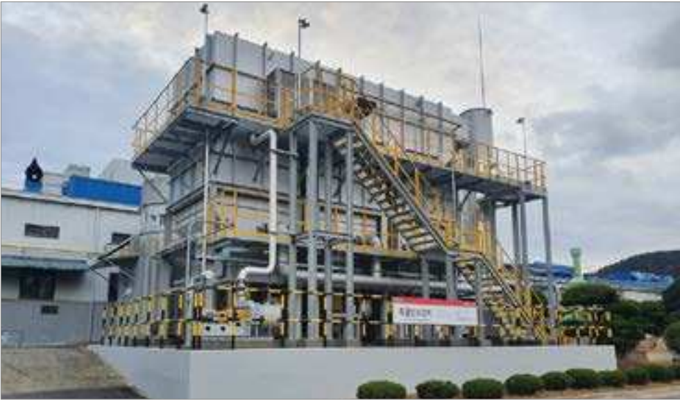
DRB Industrial’s waste gas incineration equipment
